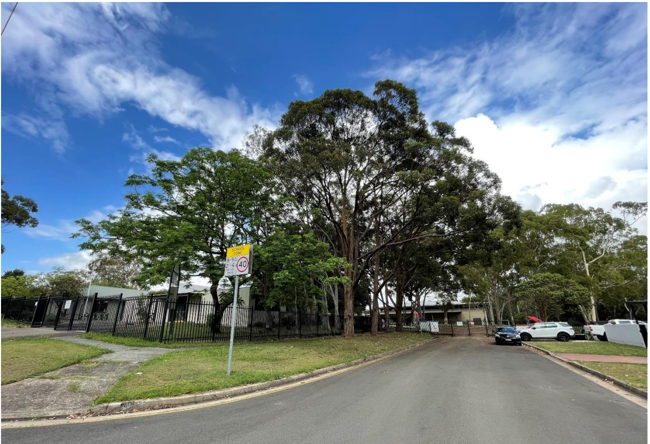
Figure 7 View of Block D from the intersection of Ashcroft and Lionel Streets (Source: EPM Projects, November 2024)
