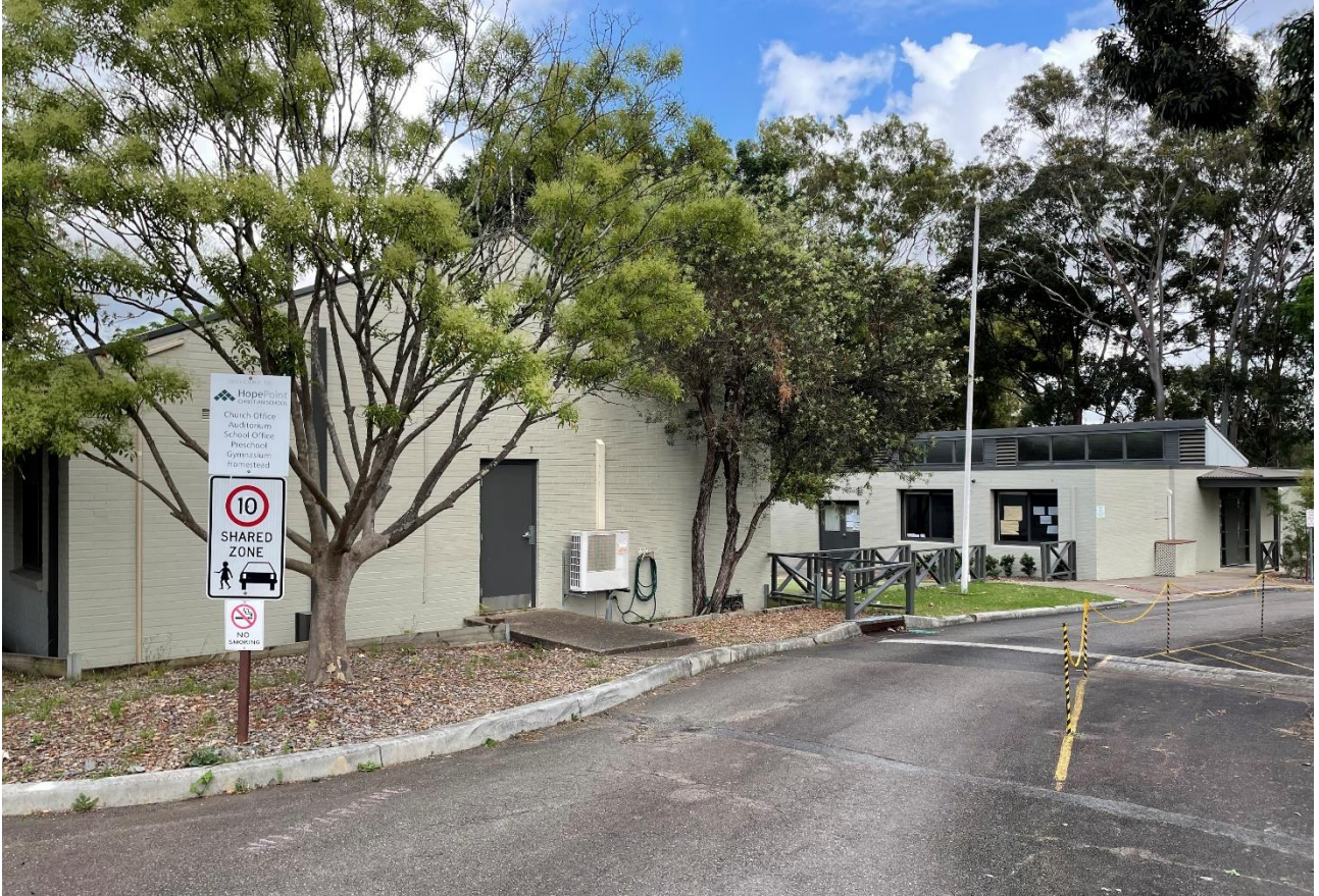
Figure 8 Blocks A and D as viewed from the pick-up and drop-off driveway (Source: EPM Projects, November 2024)
