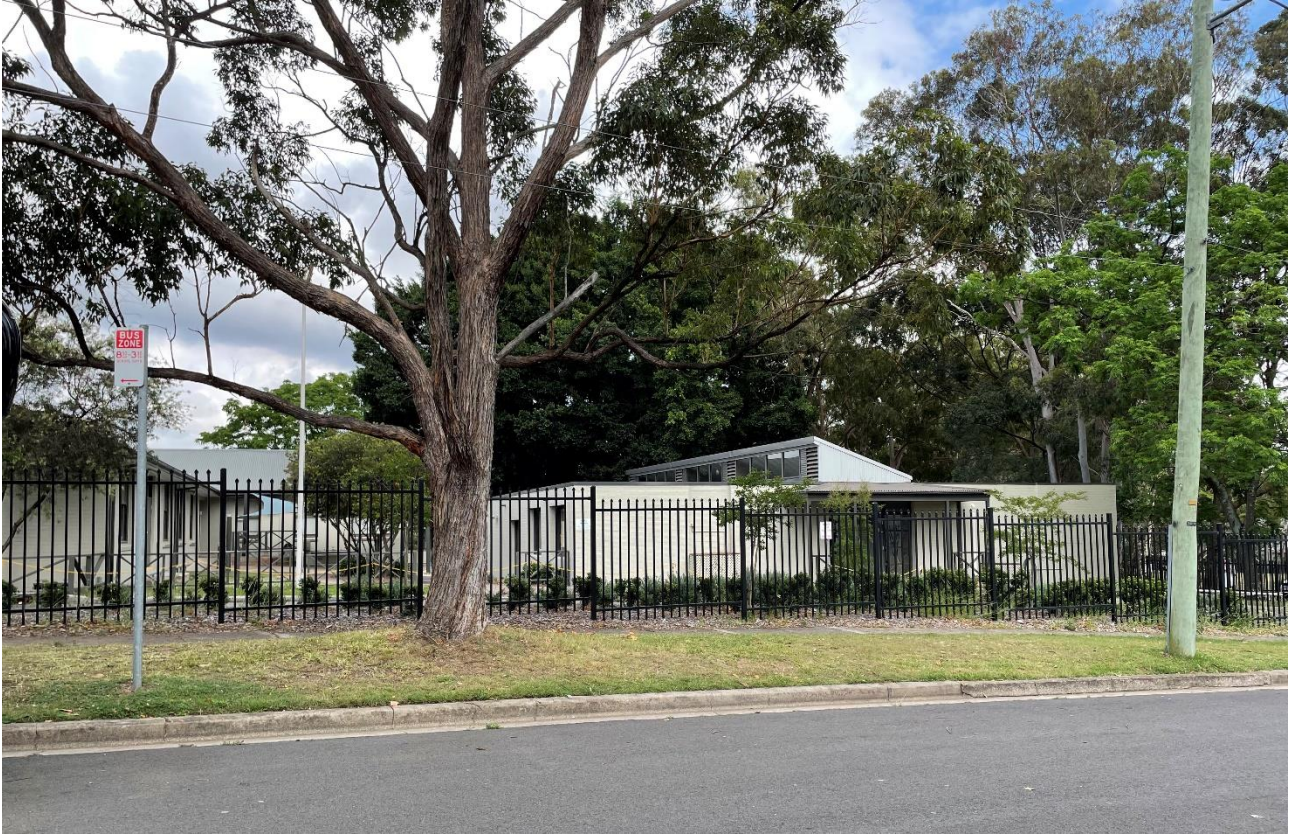
Figure 6 Blocks A and D as viewed from Ashcroft Street (Source: EPM Projects, November 2024)
